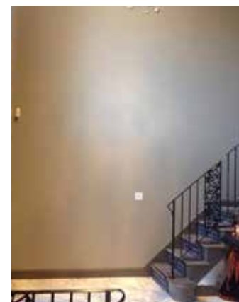
Entrance before picture
